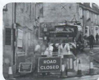
5 Repairs to streets and motorways. (4, 5)
